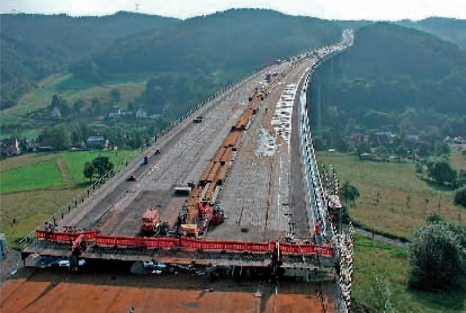
Wiehltal highway bridge, Germany.
